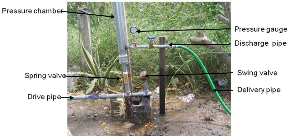
**Fig 5. Salient parts of the downdraft hydraulic ram pump**
